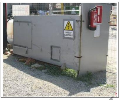
Figure 5.39: Soundproof electricity generator
