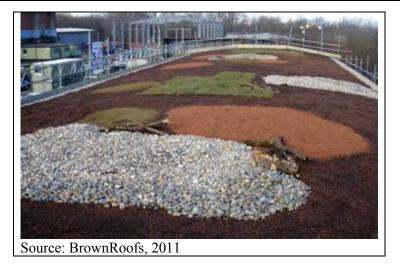
Figure 3.23: Picture of an example brown roof
