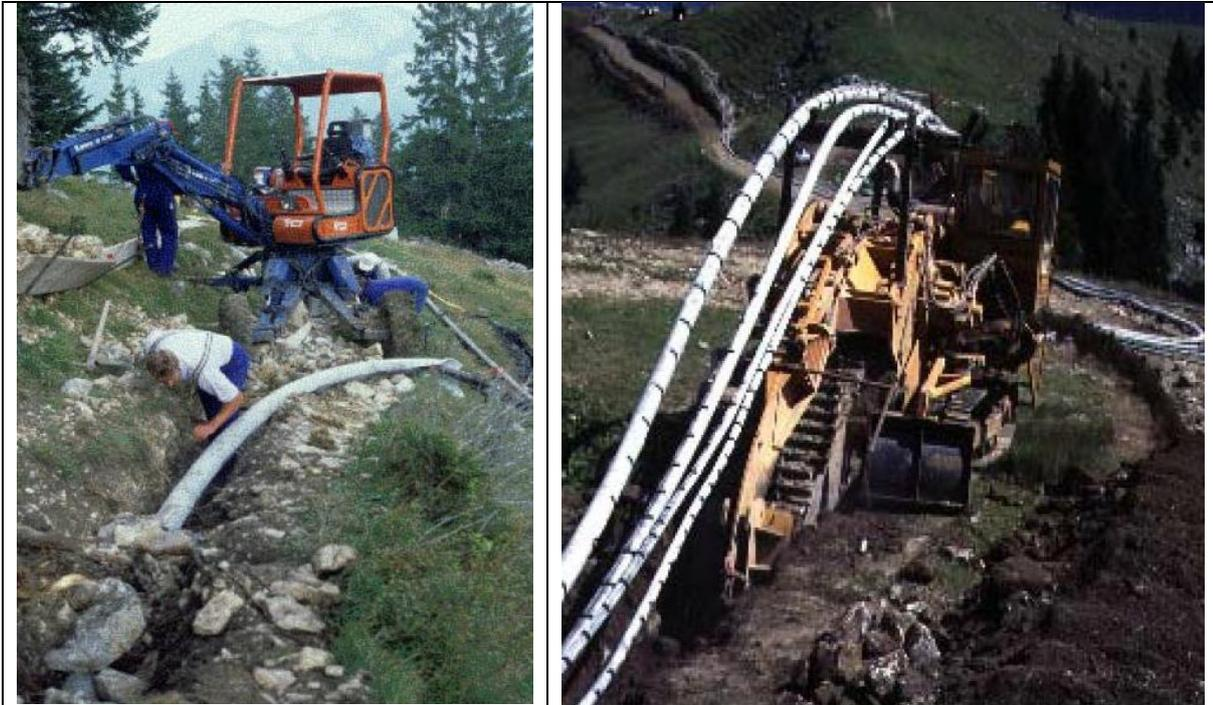
Figure 6.22: Installation of a pipe to discharge waste water down to the valley to a municipal waste water treatment plant, (BLU, 2000)
