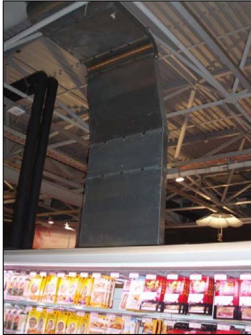
**Figure 2.46:** Air duct from a refrigeration display case to the ventilation system
