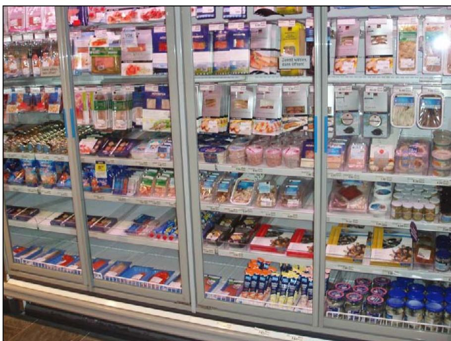
**Figure 2.45:** Vertical refrigerated display case with glass doors
