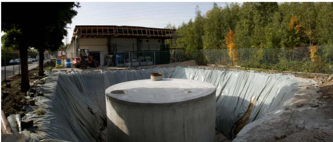
**Figure 2.121:** Rainwater collection tank (100 m<sup>3</sup>) at the Tengelmann 'Klimamarkt' in Muelheim an der Ruhr, Germany
