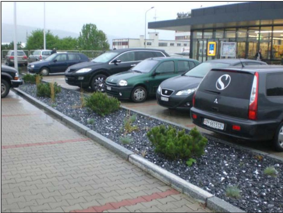
**Figure 2.122: Trench for the infiltration of rainwater of the parking area of a supermarket**
